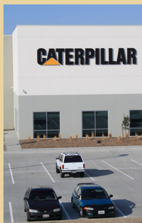
CATERPILLAR'S California Distribution Center at the Tejon Ranch Commerce Center opened in August 2012, only 8 months after the close of escrow.
